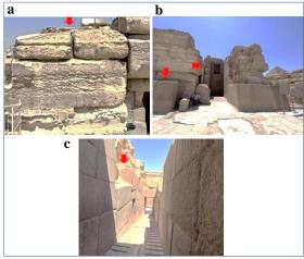
Figure (2) Shows <u>a</u>. the walls of the temple that were built of local limestone, <u>b</u>. outer and <u>c</u>. inner casing with granite blocks
