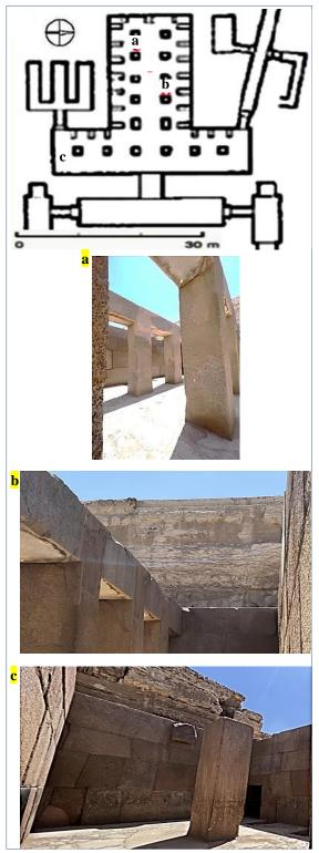
Figure (6) Shows locations of the taken photos on the plan; detachment of the surface layers, chromatic asymmetry and the appearance of dark spots as a general appearance of granite blocks
